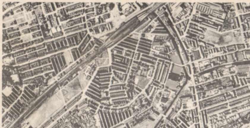
Aerial photo of Site A.
